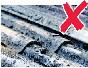
Super six asbestos roof
