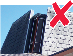
Shingle asbestos roof
