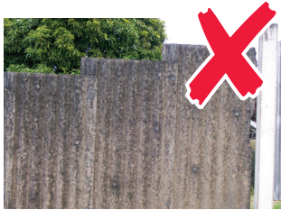
Asbestos fence
