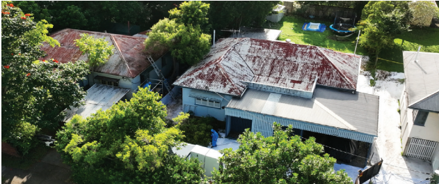
Clean up and disposal of asbestos in a residential home
