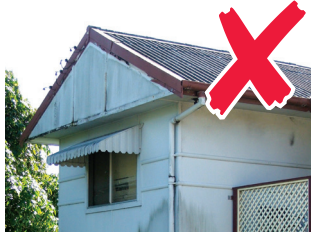
Asbestos wall sheeting
